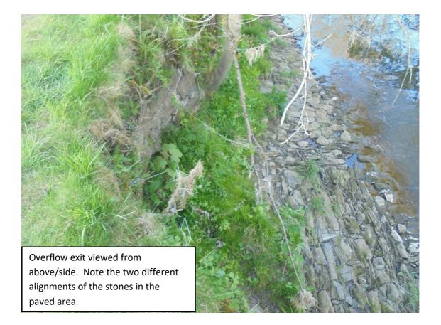
The stones underneath the overflow are aligned longways with the river flow. Either side of this area is an extensive strip of smaller stones aligned longways at right angles to the river flow.
