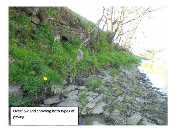
The paved area may have been an attempt to prevent erosion. The banks are very sandy in this area and easily eroded.
