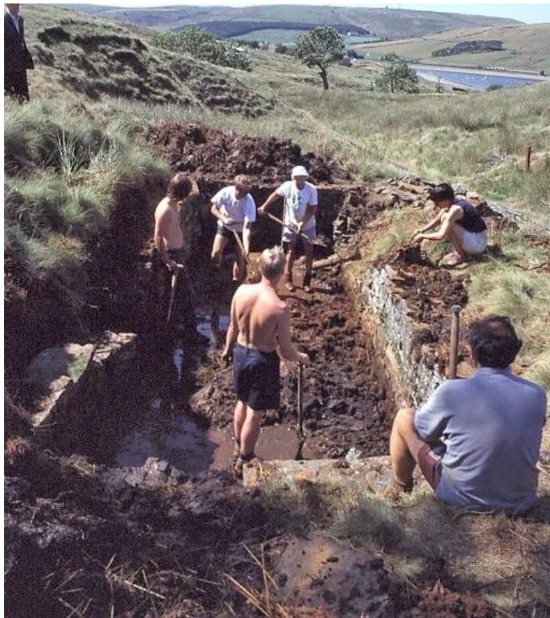
The baptistry during restoration – a very messy operation due to iron deposits in the ground water
