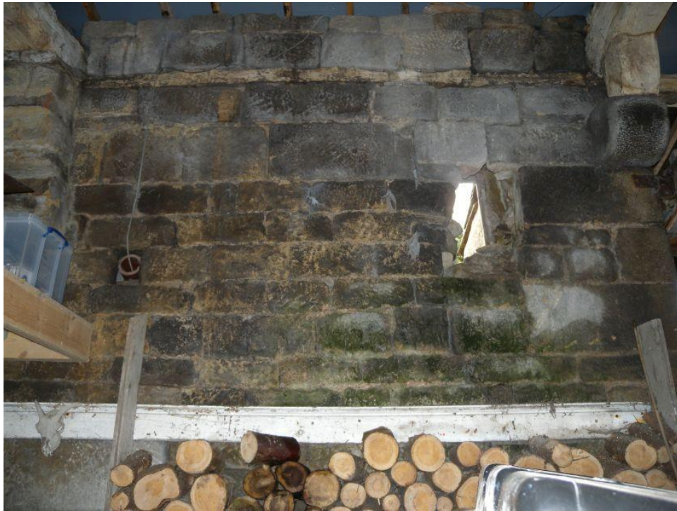
Pl. 7 North internal wall showing wall plate and projecting corbels.
