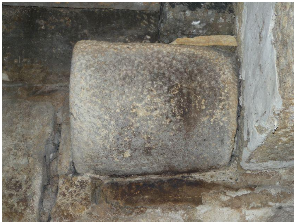
Pl. 8 Corbel detail showing picked finish
