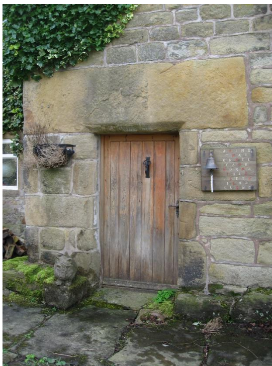
Pl. 6 Detail of side door to north elevation, note the size of the lintel
