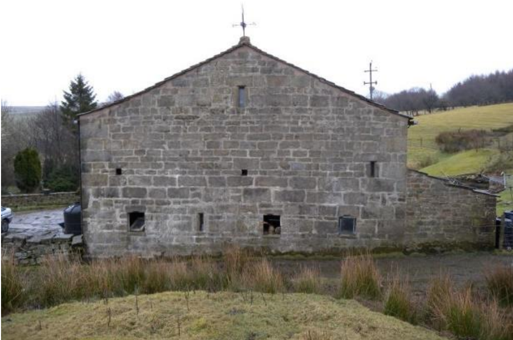
Pl. 2 West elevation, note differing depths of stone courses.
