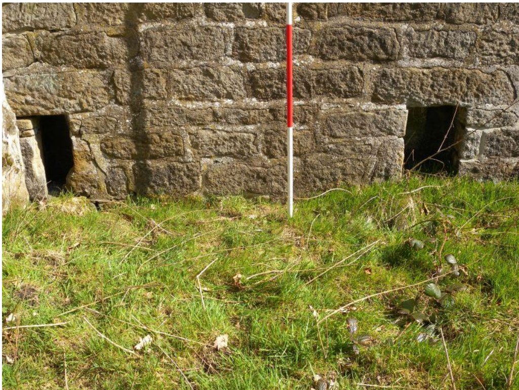
Pl. 8 External vents to east elevation; note ground level
