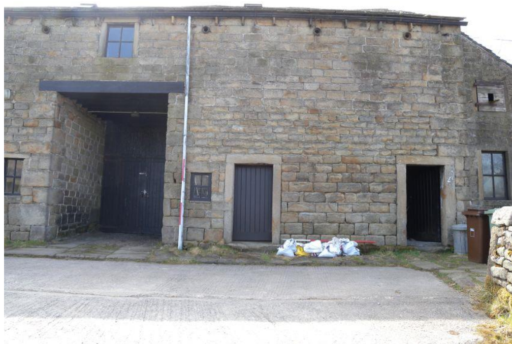
Pl. 2 North elevation (western section) note change of masonry mid-way up the wall
