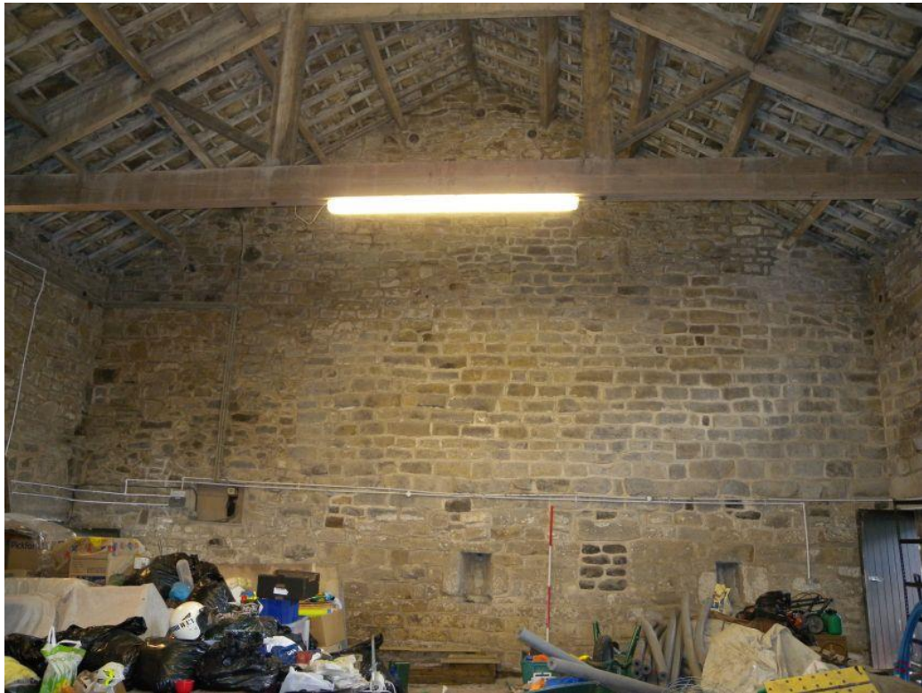
Pl. 5 East internal wall; the outline of the primary barn gable wall can be seen
