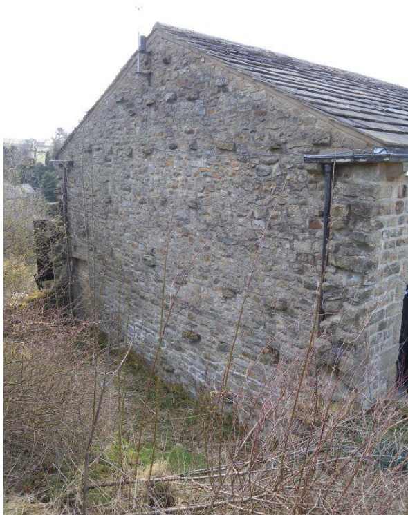
Pl. 4 South elevation showing tooththing to external walls
