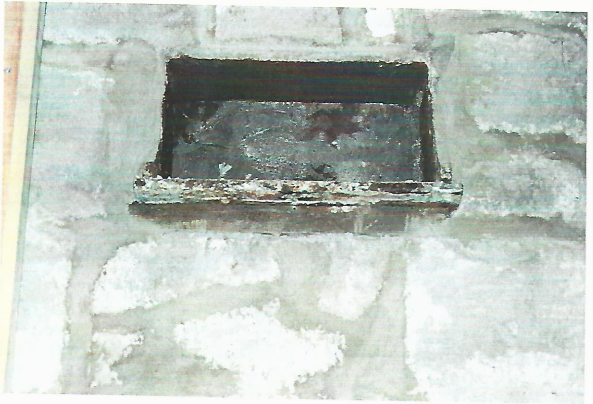
Pl. 33 First floor, cast iron bearing housing built in to external wall.
