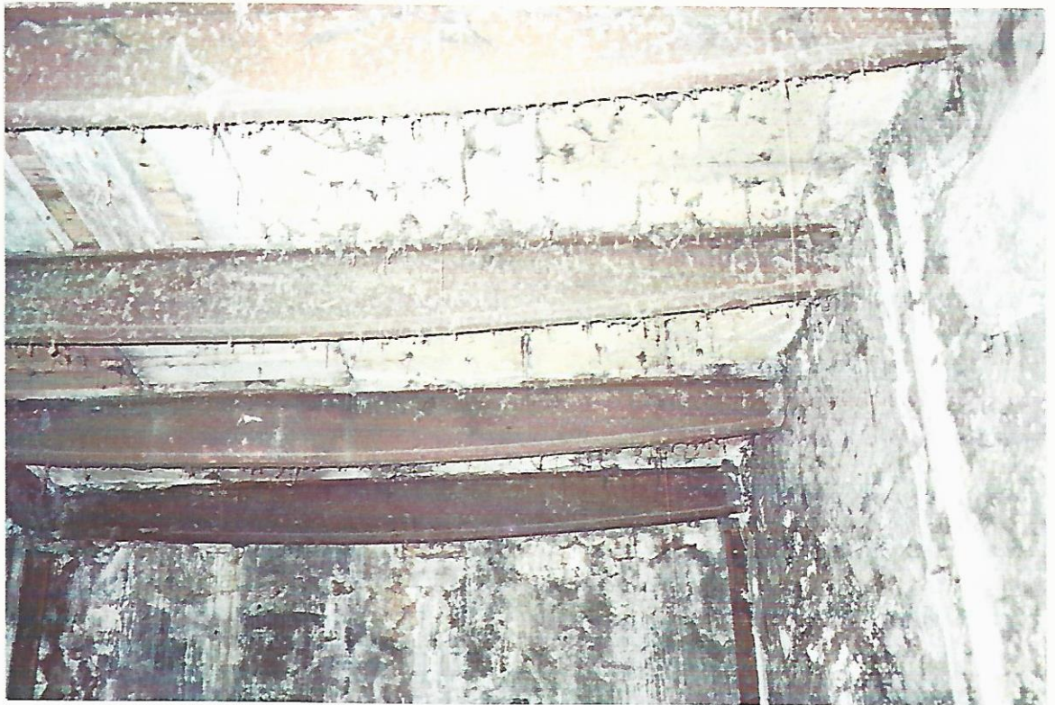
Pl. 28 First floor, cast iron beams supporting stone flagged floor above water wheel housing.
