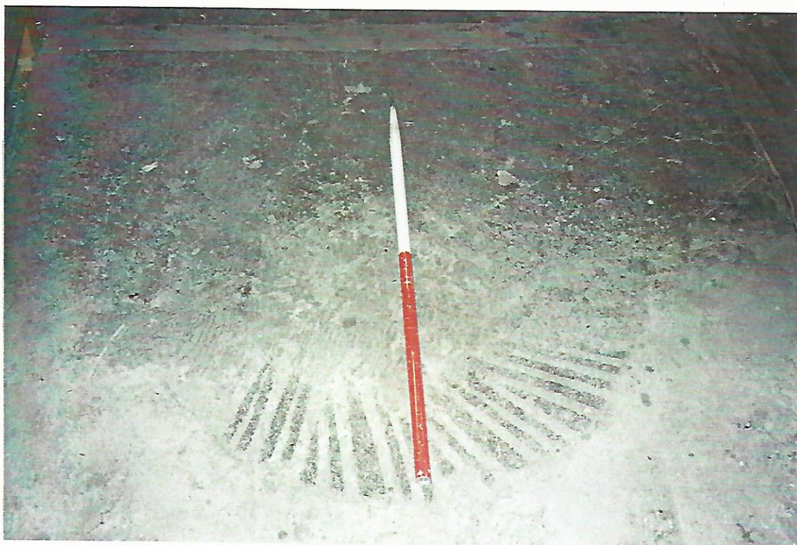
Pl. 31 First floor, upper face of millstone in cast iron millstone frame.
