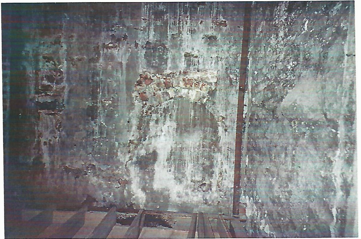
Pl. 27 First floor, entry point of leat into water wheel chamber.
