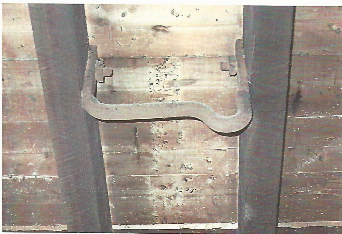
Pl. 32 First floor, iron brackets fixed over edge of millstone frame.
