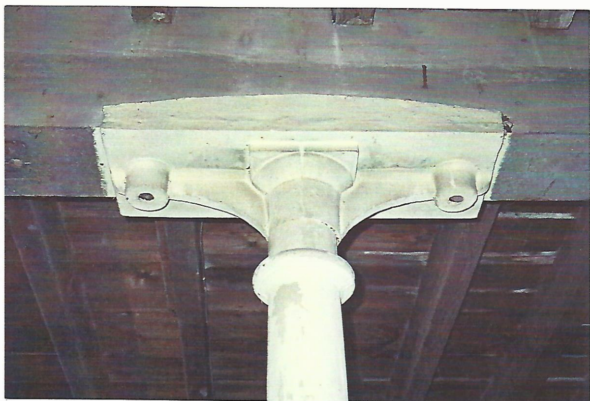
Pl. 30 Top of cast iron column used in southern section of the building.
