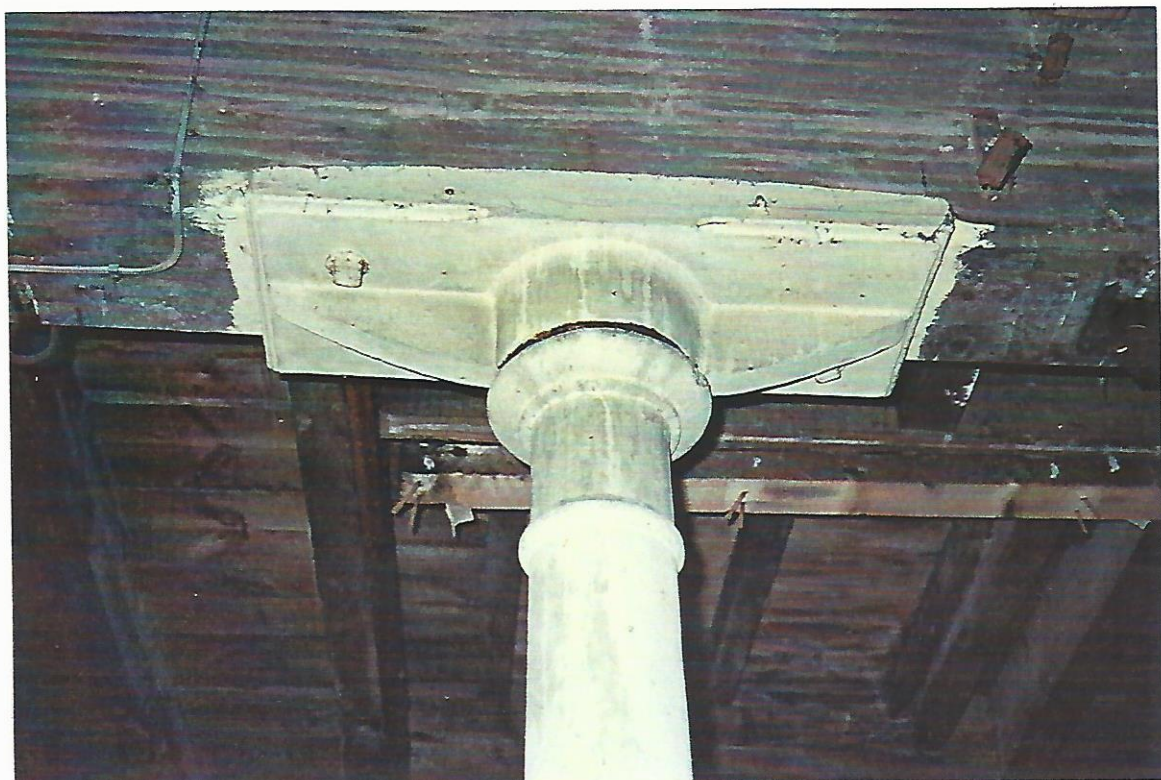
Pl. 29 Top of cast iron column used in the northern section of the building.
