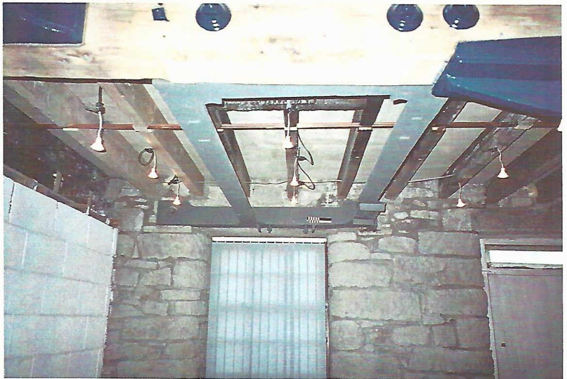
Pl. 21 Ground floor office, cast iron frame at high level.
