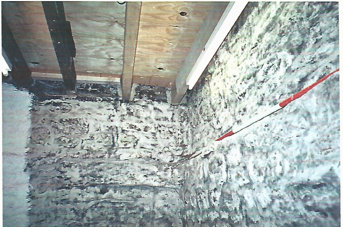
Pl. 15 Ground floor workshop with threshold of seventeenth century doorway at high level in end wall, and offset showing earlier floor level.
