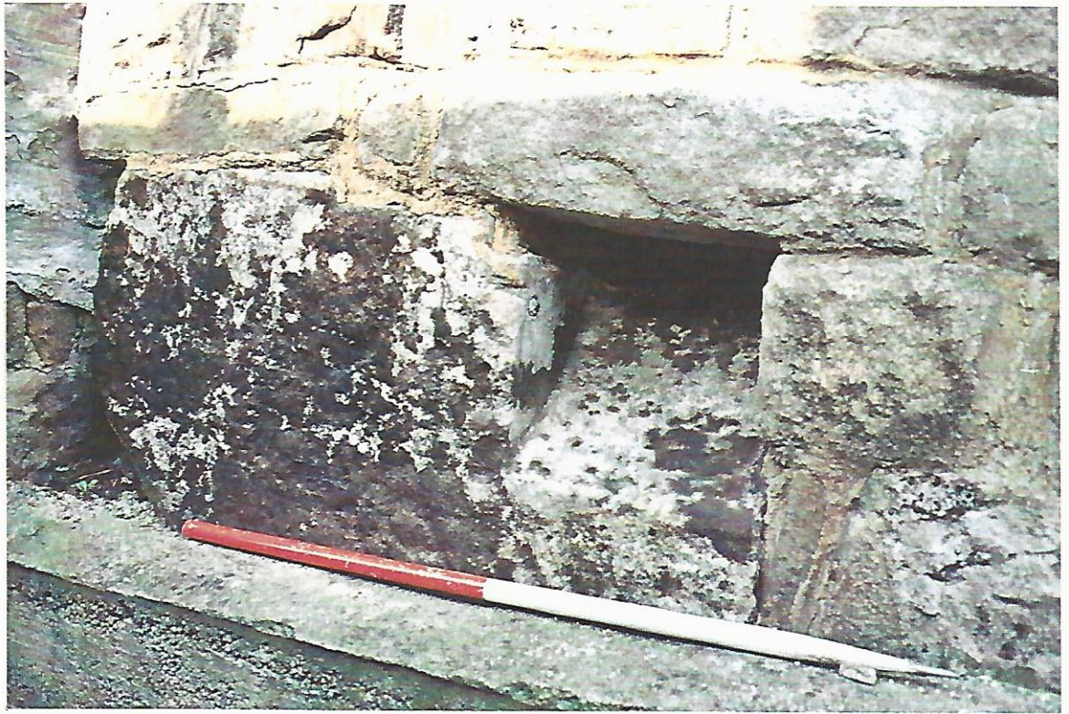
Pl. 10 South elevation of the loading bay, part of a lintel built in to the retaining wall.
