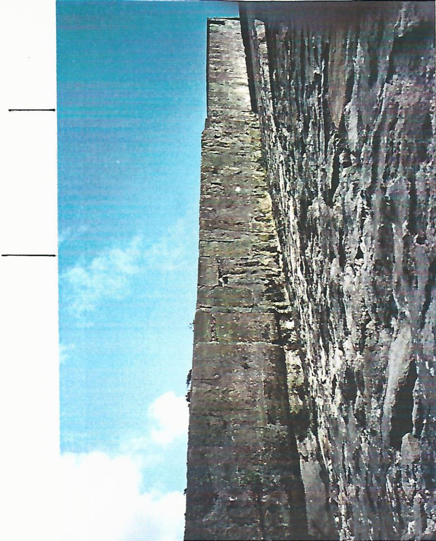
Pl. 14 West elevation showing position of offsets and edge of seventeenth century doorway.
