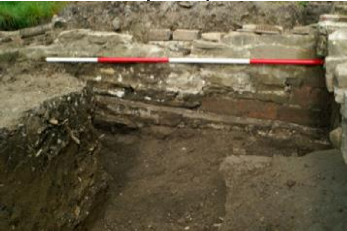
Plate 2 Northern wall showing inclined flag course on internal face.
